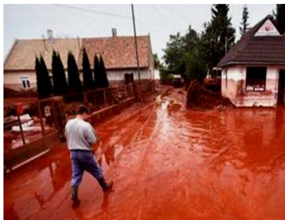
Damage caused by alkaline waste spill in Hungary, November 2010
