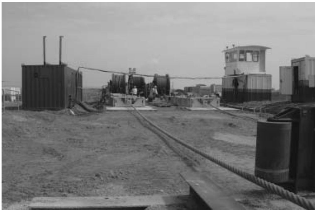
Figure 2.5. Winching operations (courtesy Van Oord)
