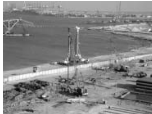
Figure 2 – Piling at top of slope
