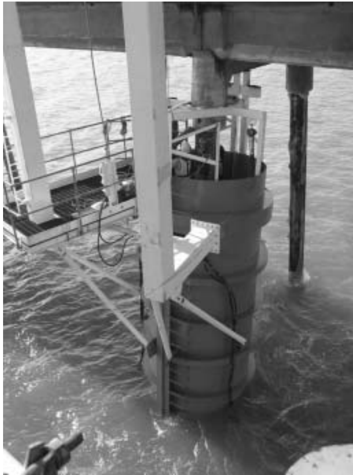
Figure 4.4. Limpet dam (courtesy John Martin Construction)
