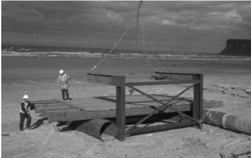
Figure 3. Deck prefabrication
