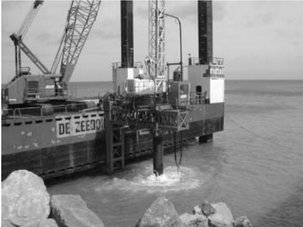
Figure 5.13. Jack-up platform used for marine piling close inshore (courtesy Edmund Nuttall)
