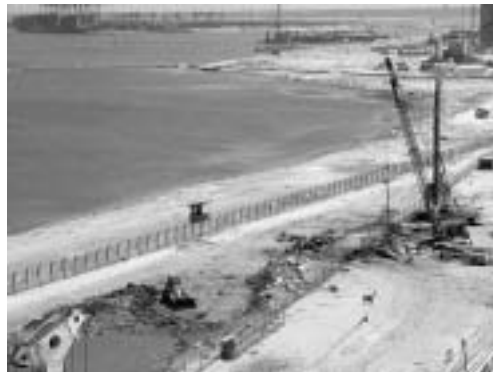
Figure 1 – New berth area
