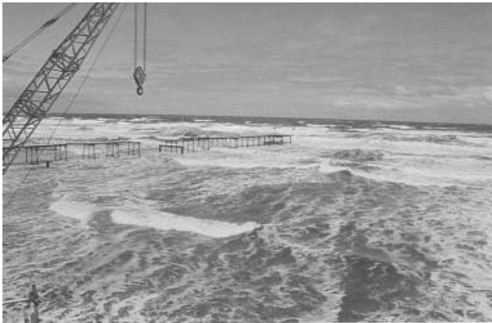
Figure 2. Storm conditions at the end of dismantling of existing pier
