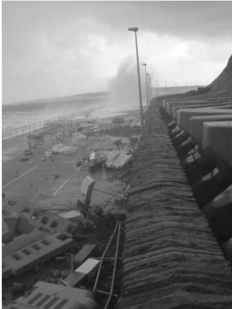
Figure 4.2. Storm damage to coastal protection site
