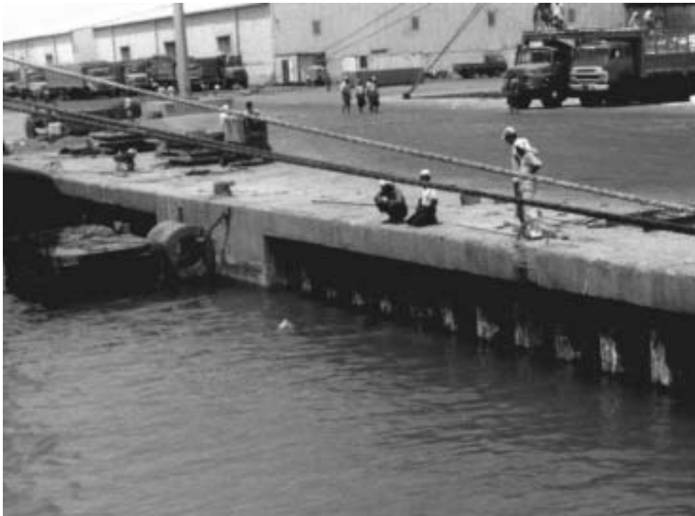
Figure 3.4. Example of different 'cultural' attitudes to health and safety Photo shows swimmer (below surface) who takes a breath and dives down several metres with a wire brush held in his mouth to then brush the rust off the sheet piles for as long as he can hold his breath before returning to the surface to catch his breath again. The whole wall was treated in this way (courtesy Alan Brampton)
