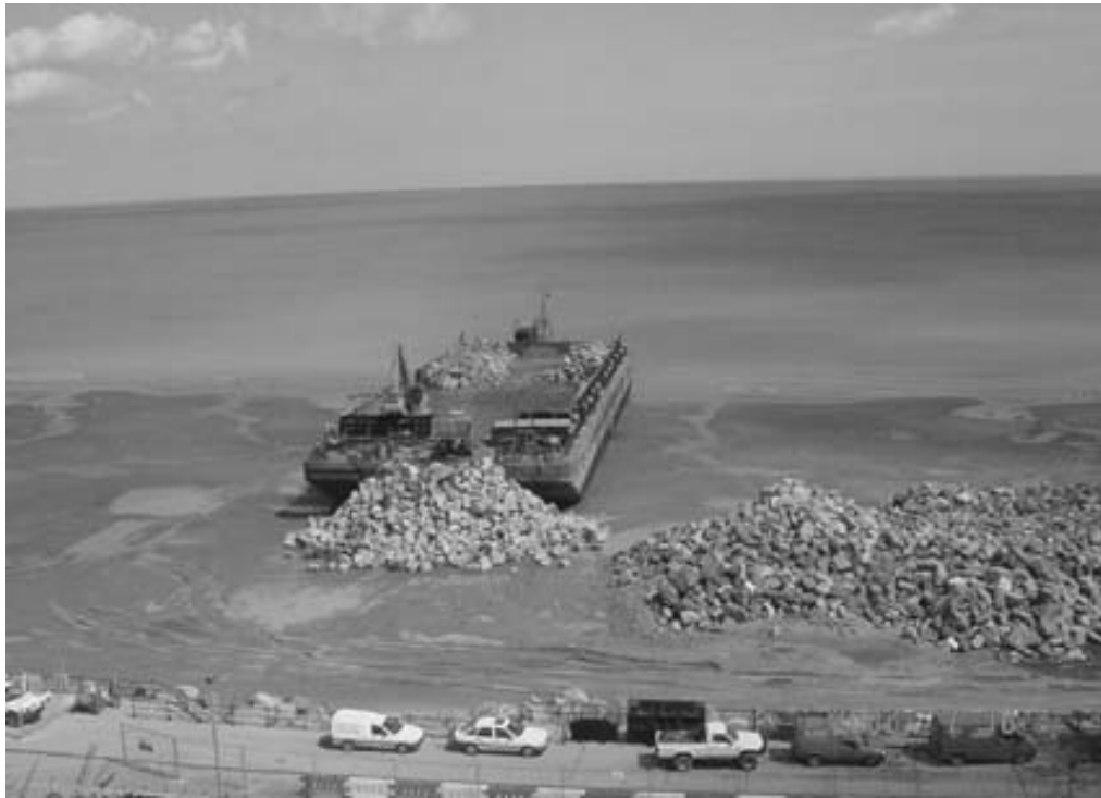
Figure 5.10. Barge used for placing rock armour sea defences (courtesy Edmund Nuttall)
