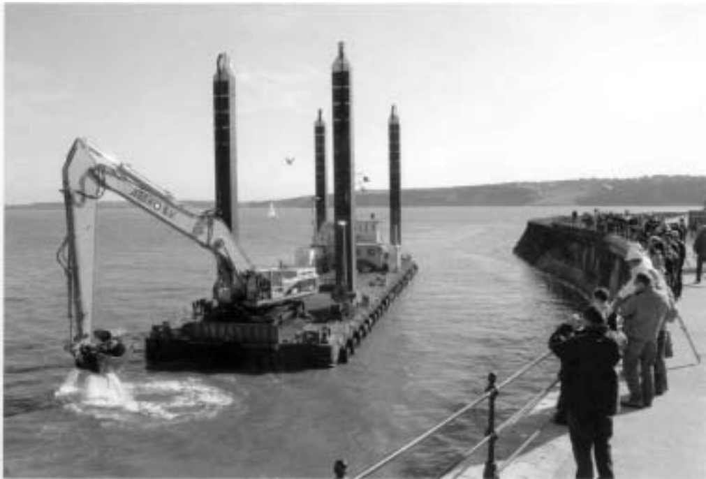
Figure 5.6. Back-hoe dredger at work close to existing seawall (courtesy Edmund Nuttall)
