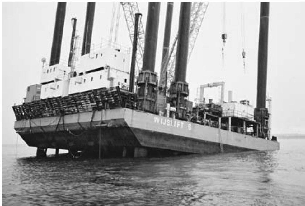
Figure 5.15. Jack-up failure (courtesy Anon)
