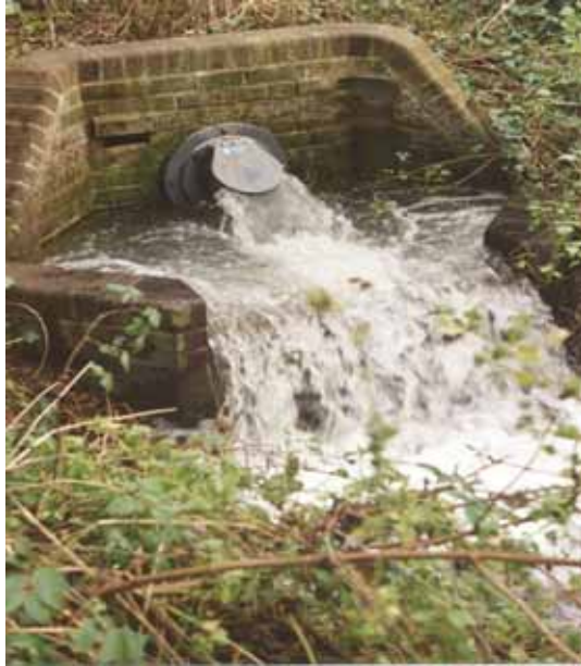
Figure 3.8 Flow augmentation of the River Darent from pumping of a Chalk borehole at Eynsford (photograph: Pauline Smedley).
