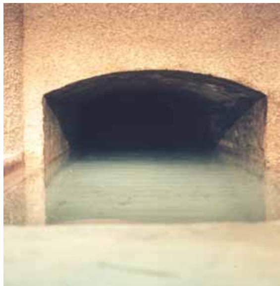
Figure 3.9 Terlingham Tunnel spring source, Folkestone is Chalk springwater discharging from the base of the formation at a rate of 65 \text{ m}^3 \text{ hour}^{-1} . The source is used by Folkestone & Dover Water Co. to supply a local drinks factory (photograph: Pauline Smedley).
