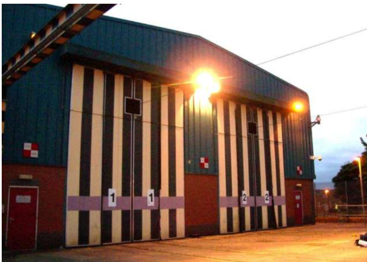
Figure 5: North-west entrance of Longsight International depot
