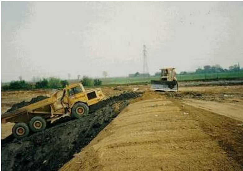
Figure F6.3 Cell Construction with Dumper and Bulldozer
