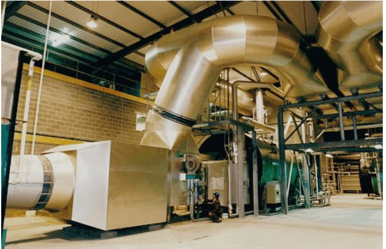
Figure F5.2 Turbine and Boiler Installation
