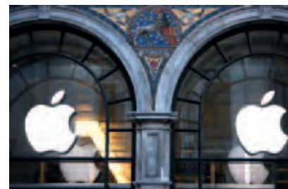
Above The world-famous Apple store, built behind the listed façade of Regent House.
