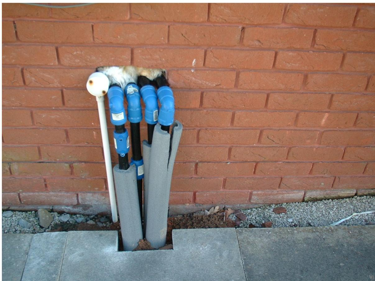
Figure 2: The two 32mm GSHP ground loops as they enter the house in parallel.
