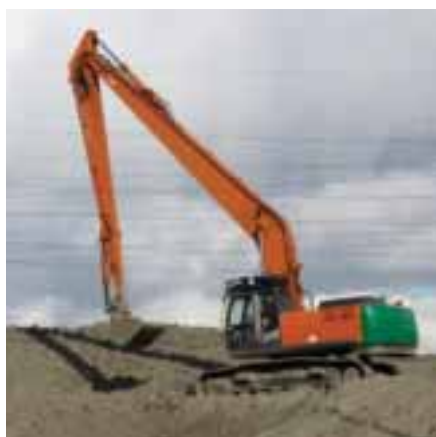
'Dig' phase of project
