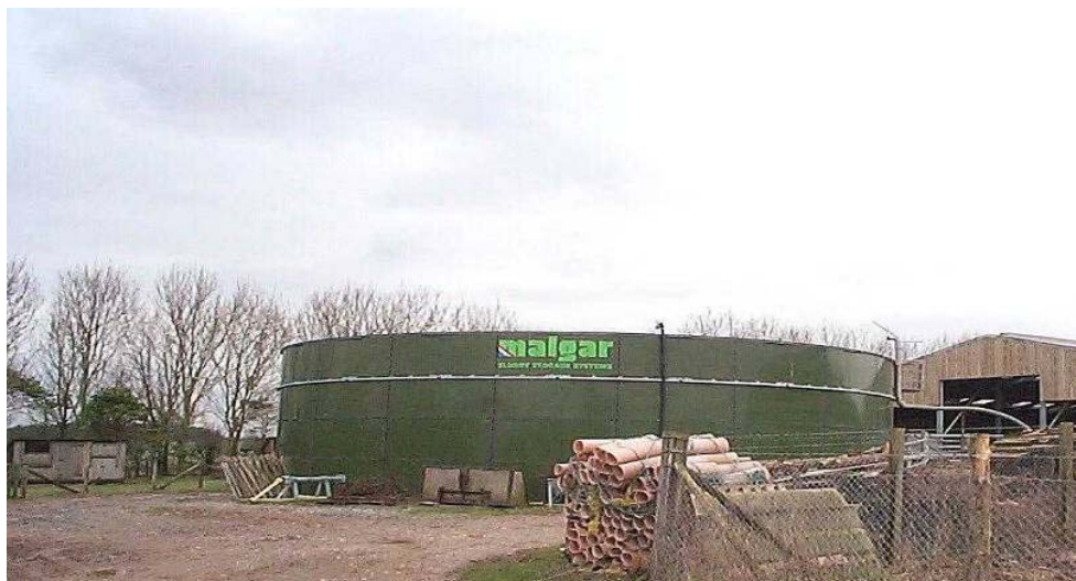
Plate 1. Example of above ground ‘tin-tank’ slurry store
