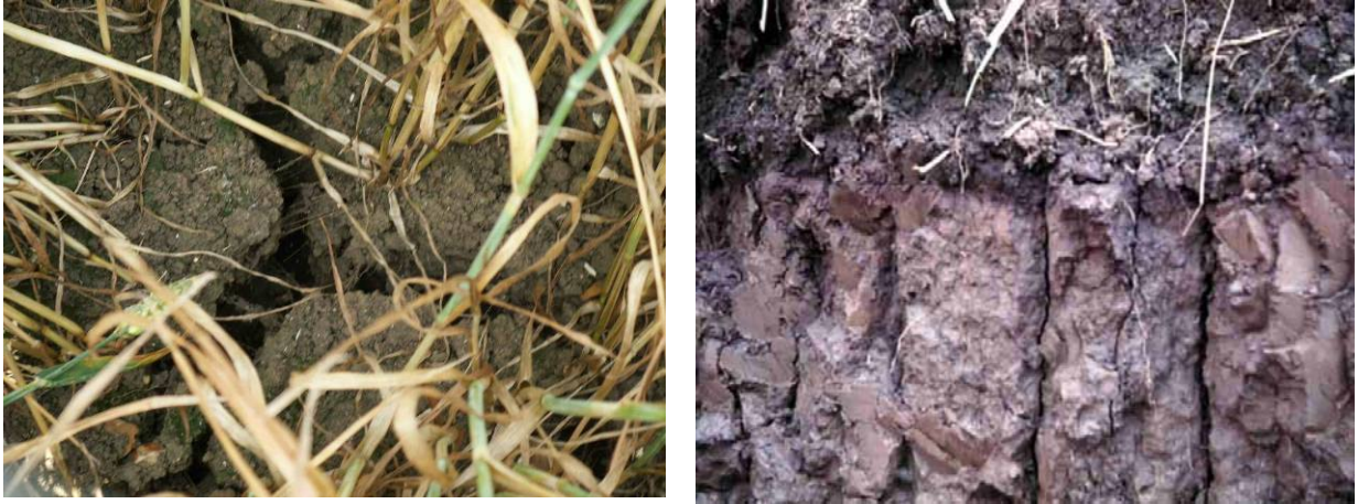
Plate 1. Cracks and fissures in medium/heavy soils.
