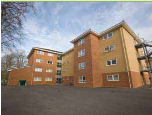
Some of the new accommodation at Pirbright
