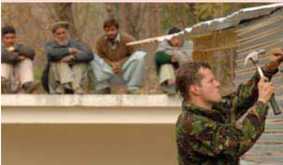
Engineers building shelters whilst a group of villagers look on
