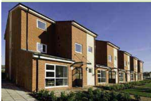
New Barracks at Tidworth Garrison
