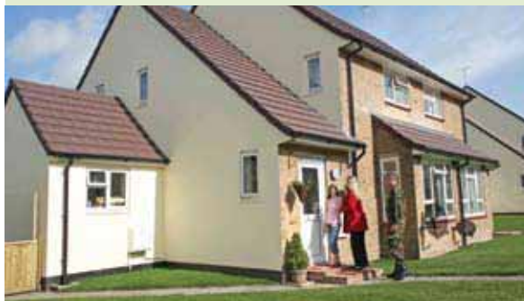
Upgraded Service Family Accommodation at Blandford Camp
