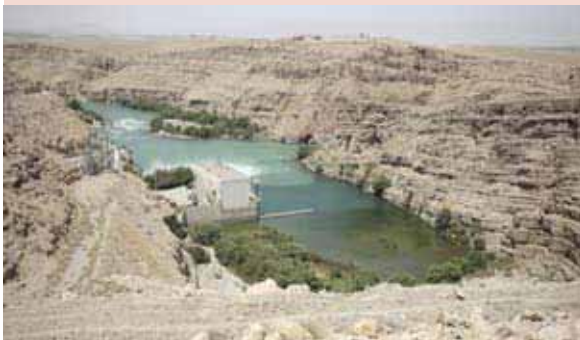
The Kajaki hydroelectric dam, Helmand province, southern Afghanistan
