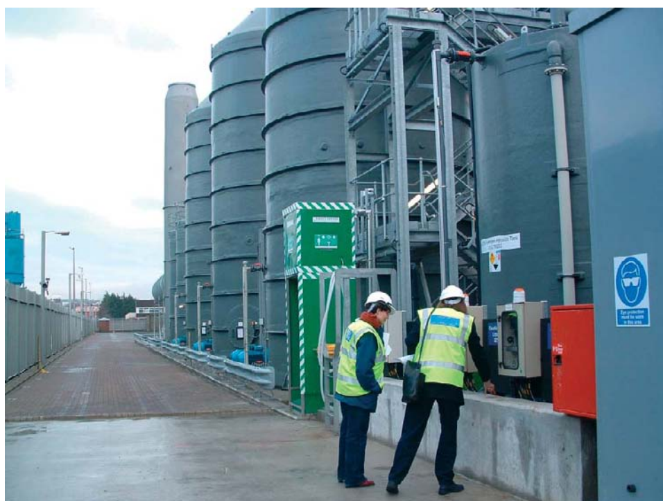
Site visit to treatment works (© CHaPD London)
