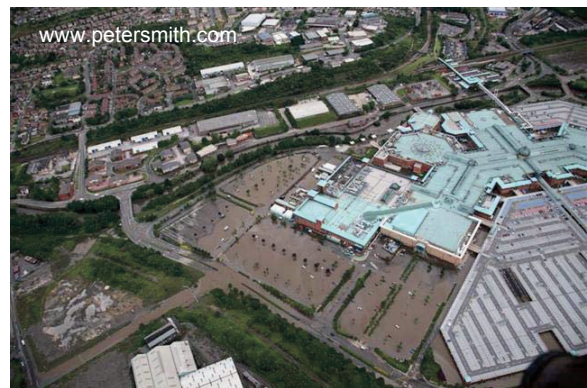
Meadowhall under siege from floodwaters
