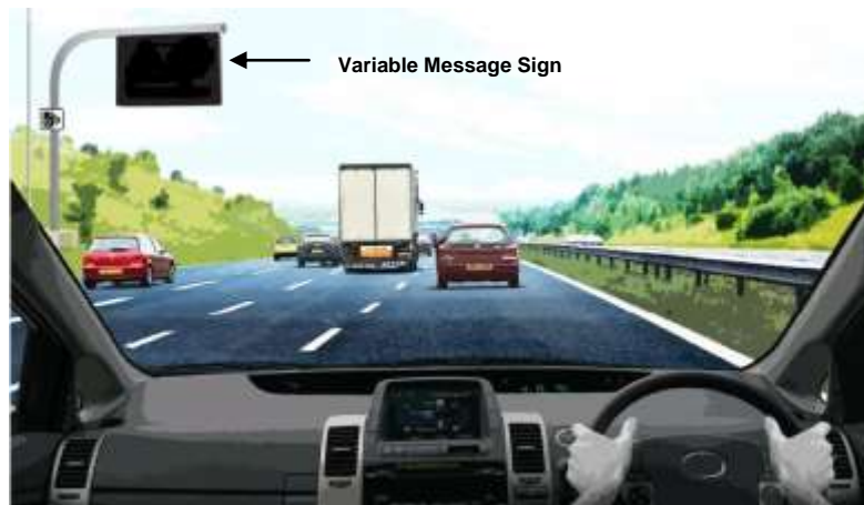
Figure 4B: Illustrative M1 J39 to J42 Managed Motorway scheme section operating in normal motorway conditions with a blank verge mounted variable message sign
