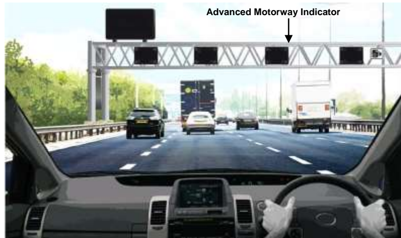
Figure 4A: Illustrative M1 J39 to J42 Managed Motorway scheme section operating in normal motorway conditions with blank advanced motorway indicators and blank gantry mounted variable message sign
