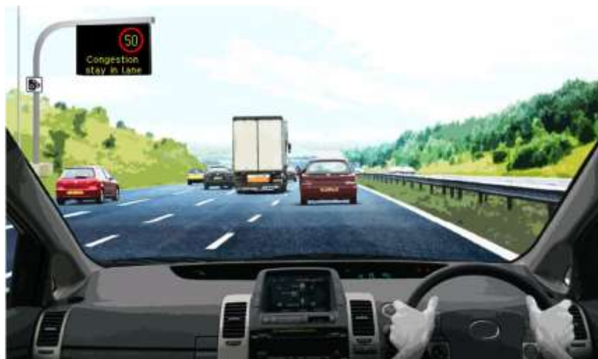
Figure 4D: Illustrative M1 J39 to J42 Managed Motorway scheme section operating with variable mandatory speed limits and information for road users.
