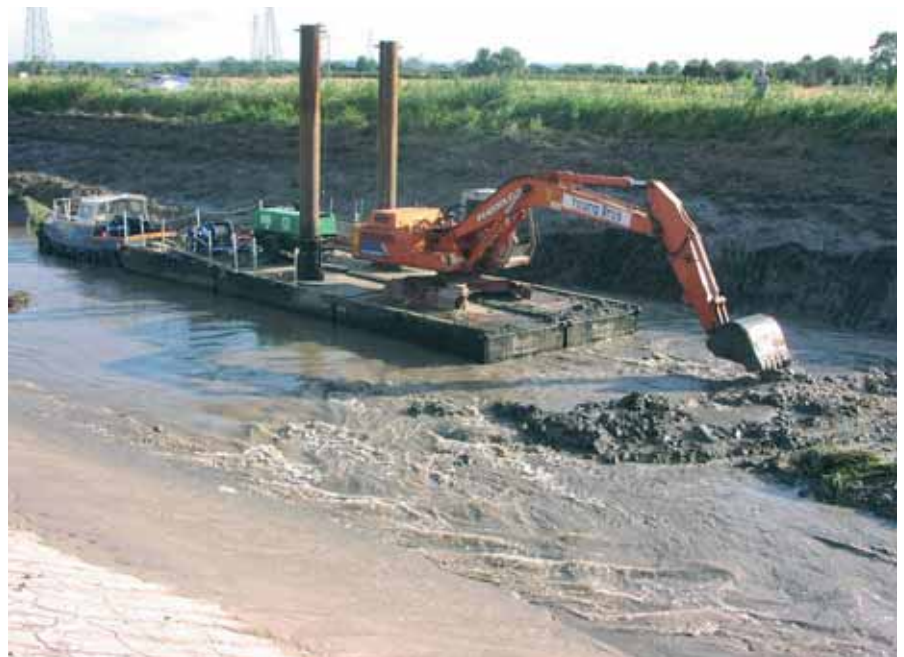
↑ Past dredging of the tidal Parrett near Bridgwater – we will study natural processes to inform the need for future operations
