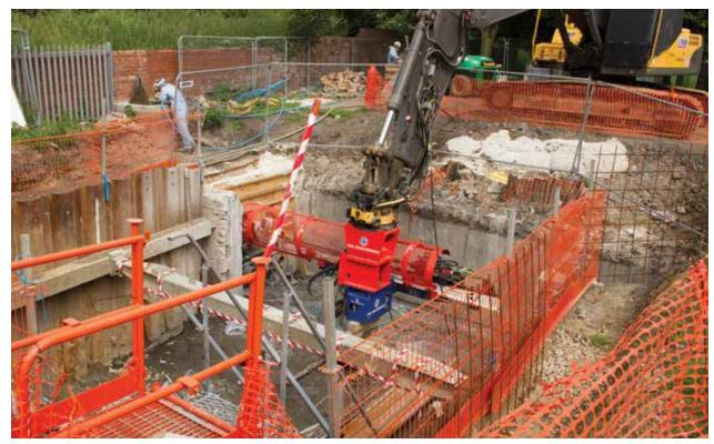
Horizontal drilling operation to enable a former colliery subway in South Yorkshire to be grouted.
