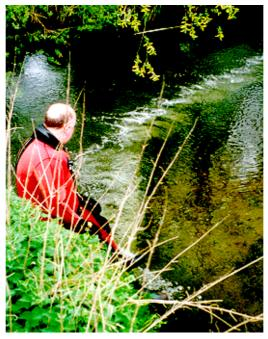
Plate 3.12 Bubble curtain laid across a small stream
