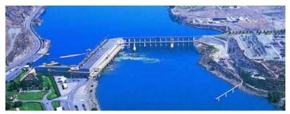
Plate 3.14 Rocky Reach dam with the powerhouse on the left and the bypass pipe in the bottom right (Chelan County PUD).
