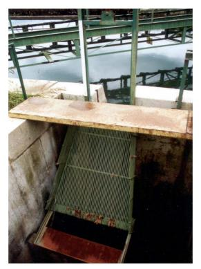
Plate 7.3 A Wolf trap photographed at Halsou, France. Water is strained through a set of parallel rods or slats that run along the length of the channel. These are spaced at about 6mm apart, allowing water to pass through, while fish are flushed along the slats and into a holding tank at the downstream end.
