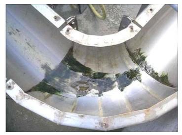
Plate 3.8 A sharp bend in this fish return gulley demonstrates the issue of biofouling where uneven joints have encouraged algal growth, causing a flatfish to take cover there. A smooth surface or exclusion of light would have prevented this.
