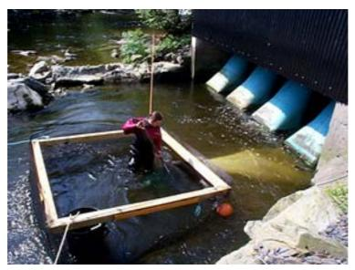
Plate 7.1 Total flow netting at the draft tube of a small hydropower turbine. Here, fish enter a live-car at the cod-end of the net to facilitate removal and to reduce the likelihood of net-induced injuries .
