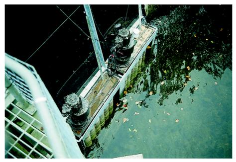
Plate 3.4 Rotary Disk Screen at Testwood Raw Water Intake, R. Test, Hants
