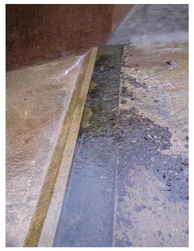
Plate 3.15 Eel bypass trough at Backbarrow hydropower scheme, R. Leven, Cumbria (Spiby, 2004).
