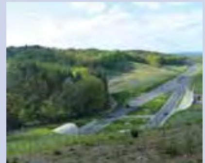
View north from above the new the tunnel
