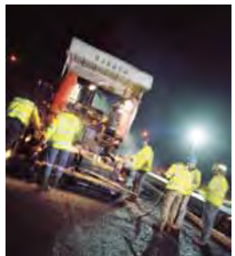
Night-time resurfacing of the M1, at Junction 19
