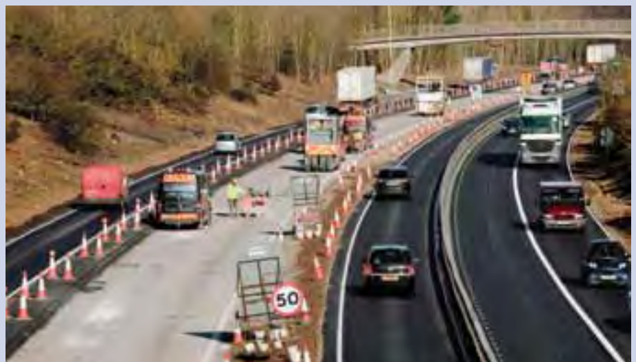
Contraflow in place to minimise lane closure
