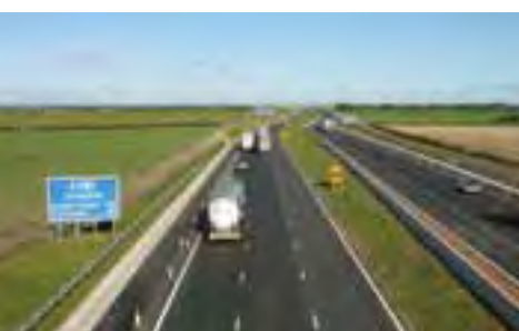
A1(M) Dishforth Rainton Bridge
