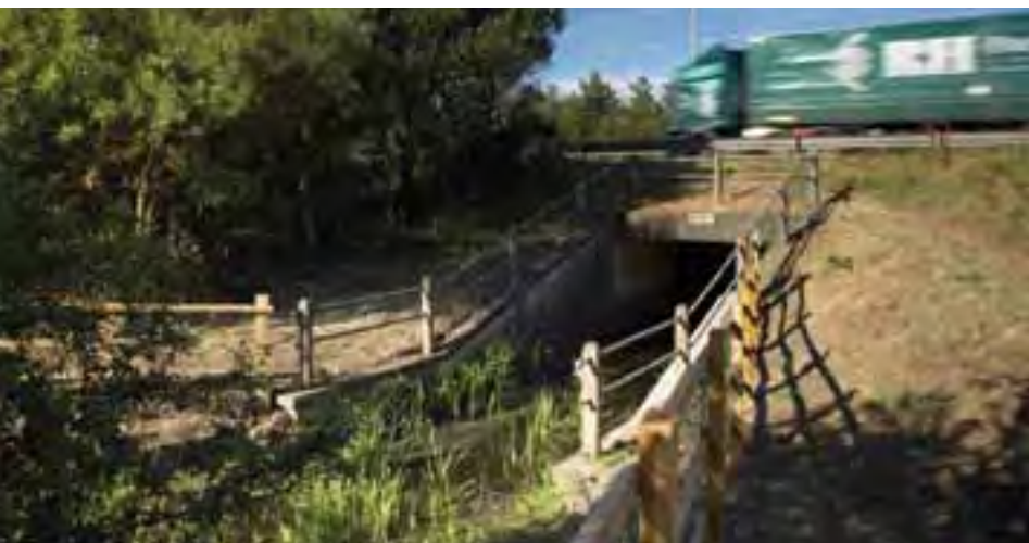
Stream running under the new road
