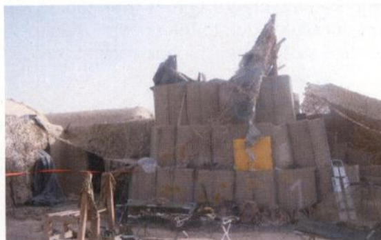
Fig 1-8 Damaged Sangar at PB Bahadur
