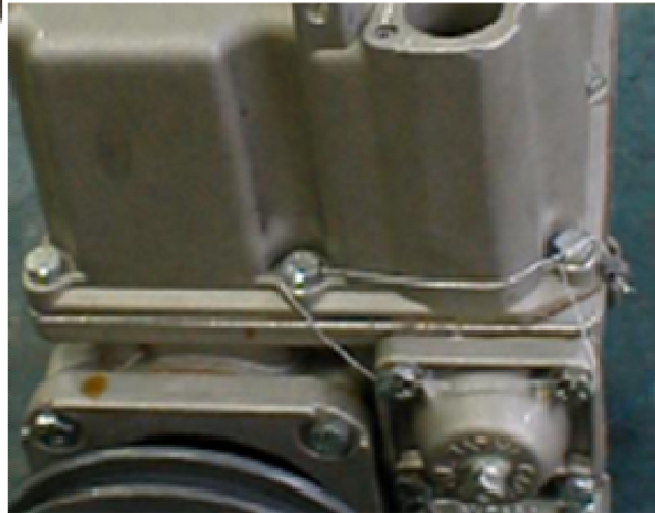
Figure 5b GPU-90 Pumping Unit Sealing
