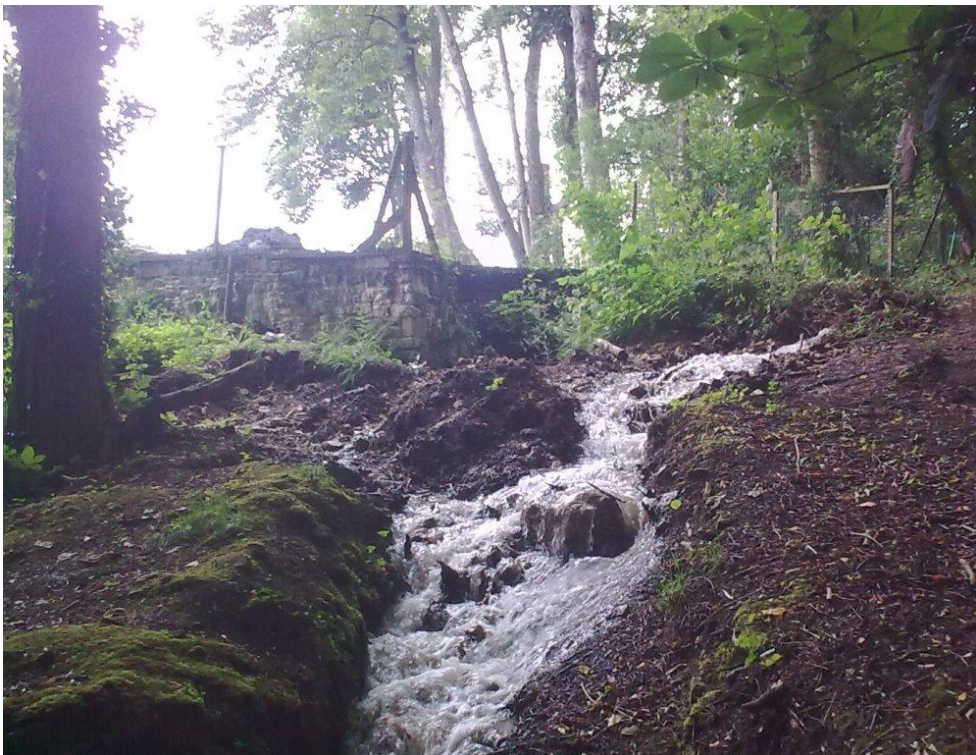
Photographs showing the temporary spillway arrangements
