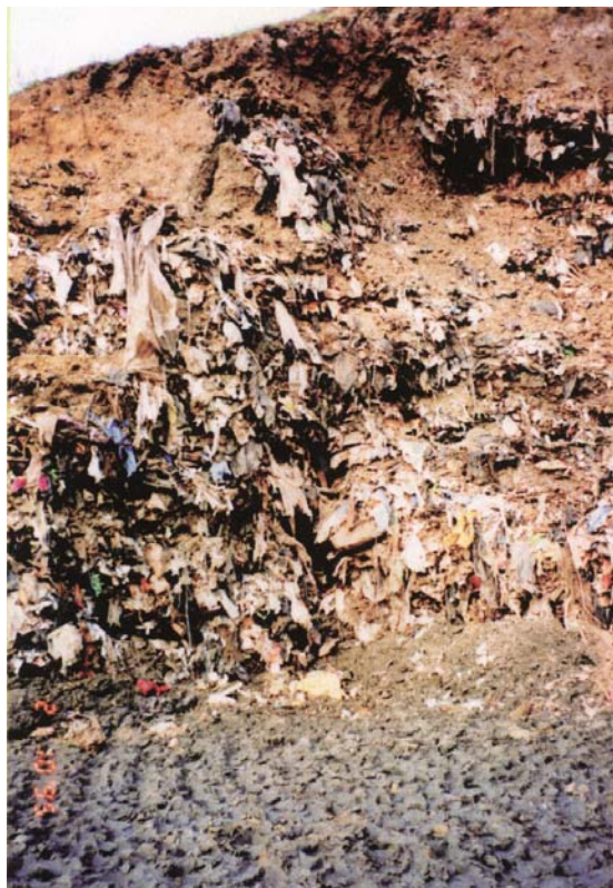
Figure 4.10 Steep slope in waste showing the reinforced nature of the material
