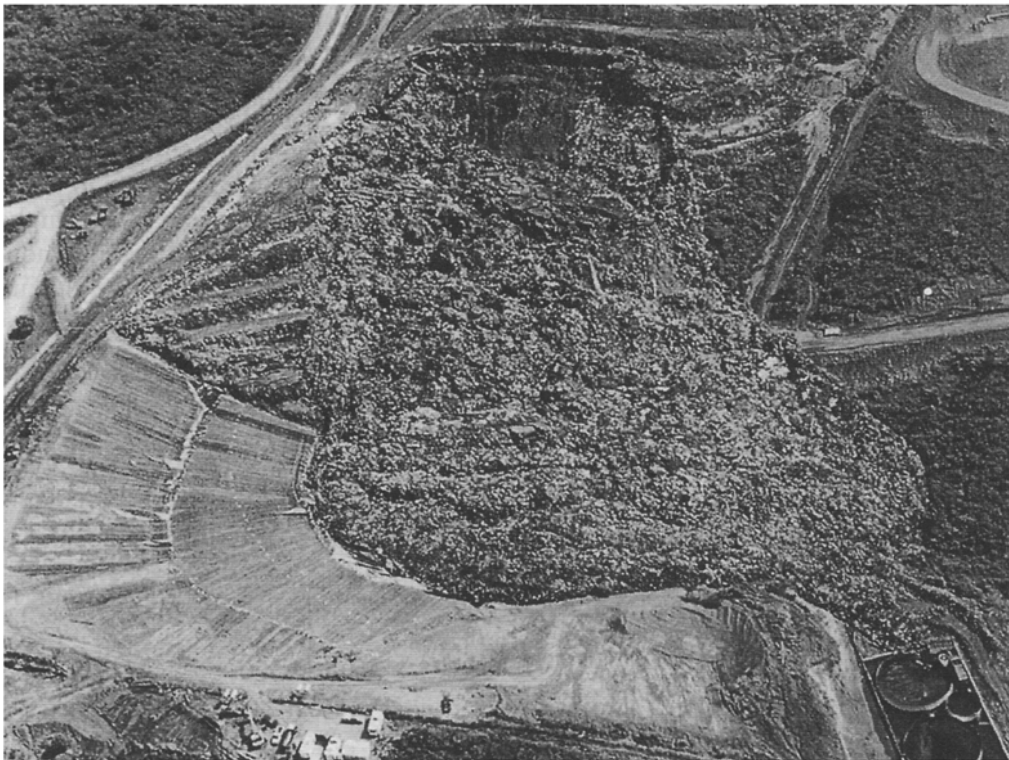
Figure 11.11 Bulbul Drive landfill shortly before and following failure (Brink et al. 1999)
