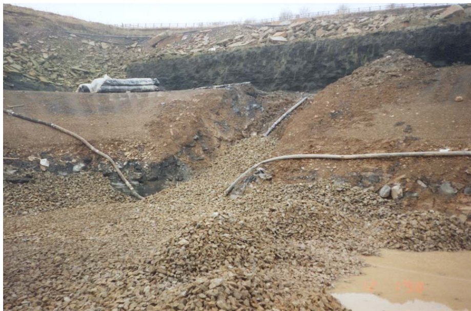
Figure 4.7 View of drainage works to control local groundwater
