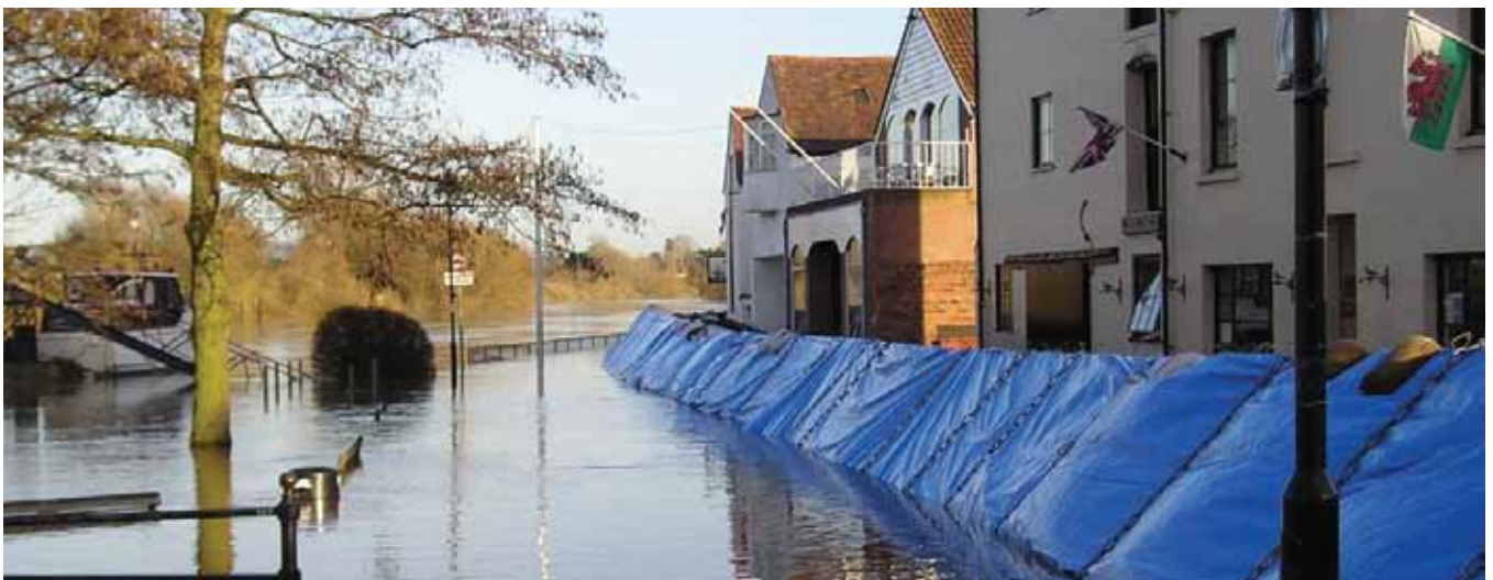
↑ Temporary flood defences, Upton upon Severn
