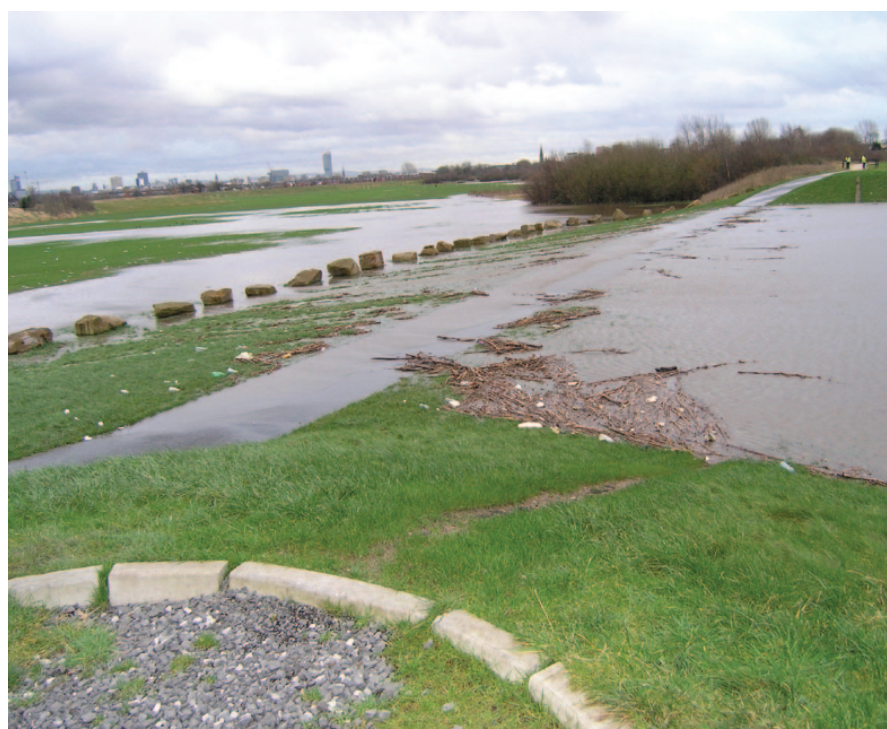
↑ Flood storage Salford Basin in operation
