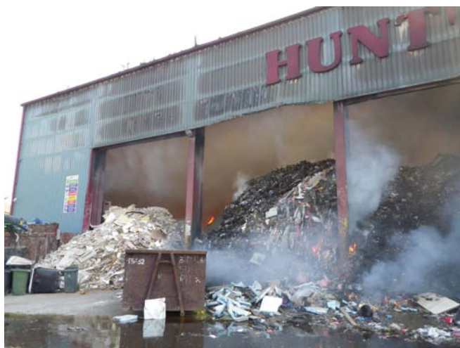
Figure 4: Mixed waste types were present on site, Dagenham, London (© London Fire Brigade 2012)
