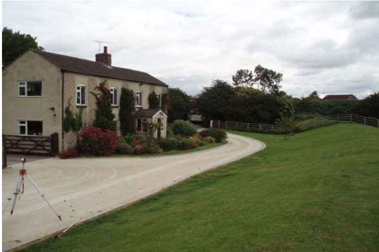
Plate A7.4 Existing Embankment around Grounds Farm in Reach 6
