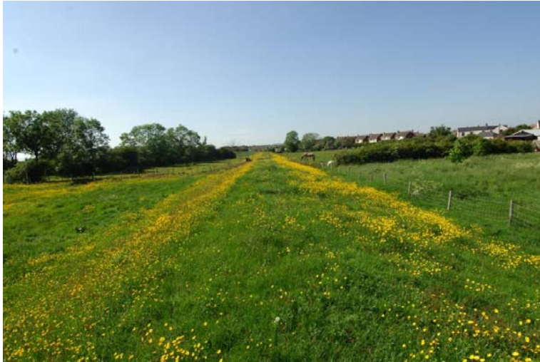
Plate A7.1 Existing Embankment in Reach 1, West of Sawley Village
