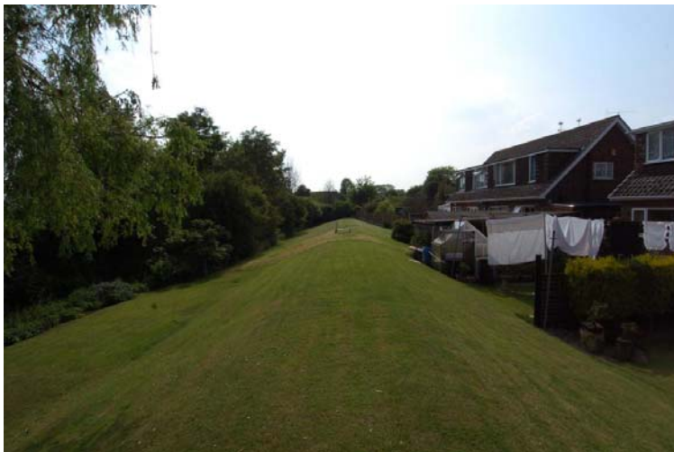
Plate A7.5 Existing Embankment in Reach 8 at Newbery Avenue
