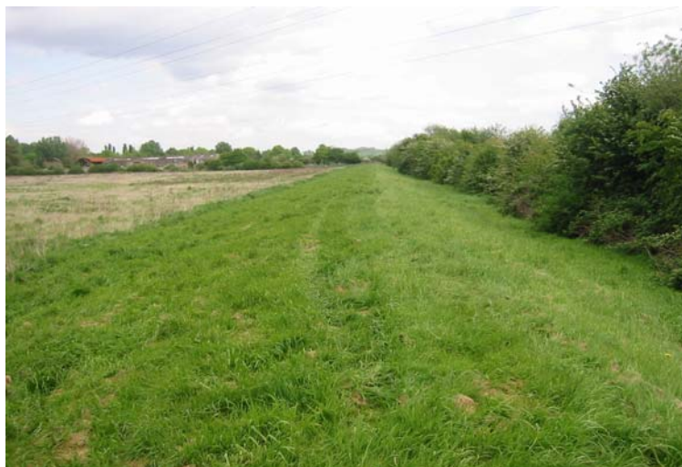
Plate A7.6 Reach 9 adjacent to New Sawley Brook
