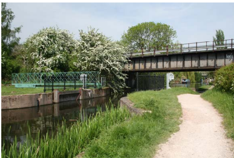
Plate A7.3 Existing Sheetstores flood gates in Reach 5
