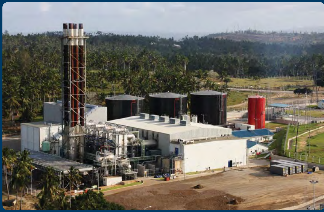
EAIF/PIDG (Rabai Power Plant, Kenya, 2012).
