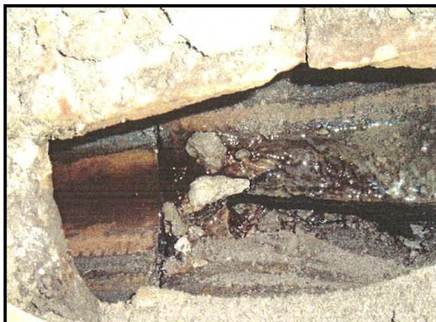
Figure 1 – Broken drain
