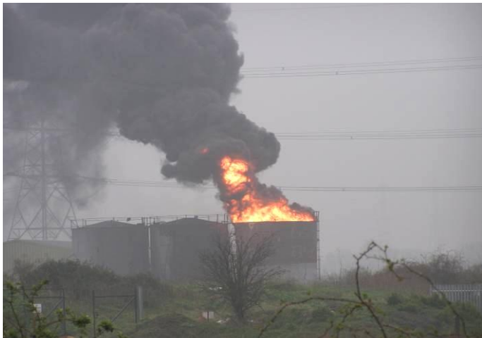
Figure 1 - Tank 4 on fire
