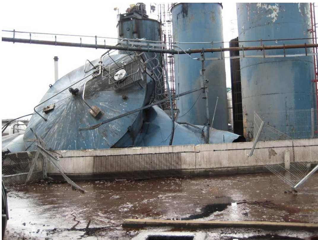
Figure 1 - Collapsed tank and spillage.
