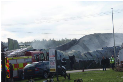
Figure 2 – Incident 3 collapsed transfer building
