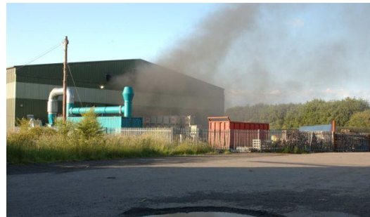
Figure 1 – incident 2, smoke exiting building
