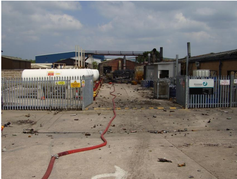
Figure 1 - Damage and aerosol debris on roof of nearby building
