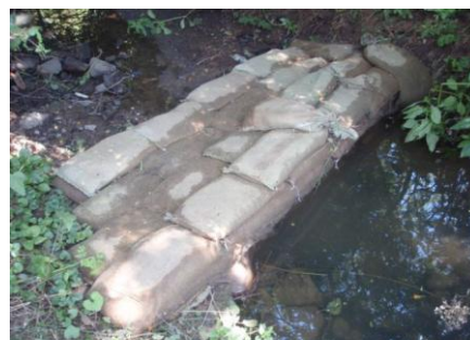
Figure 3 – Fleet Beck dammed using sandbags and booms.
