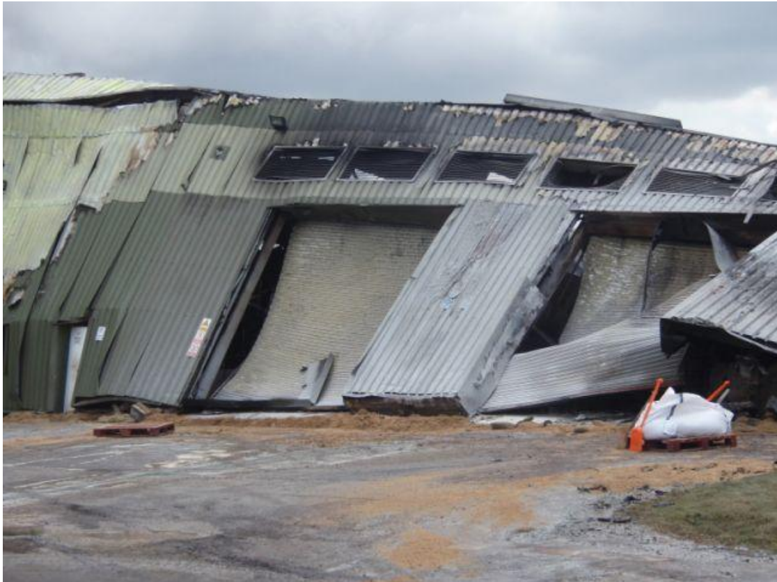
Figure 3 – collapsed building and emergency sand bagging along bottom of the door.
