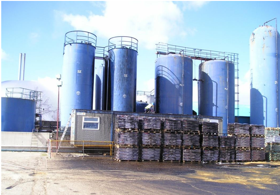
Figure 1 - Bulk oils storage tanks and oil spillage
