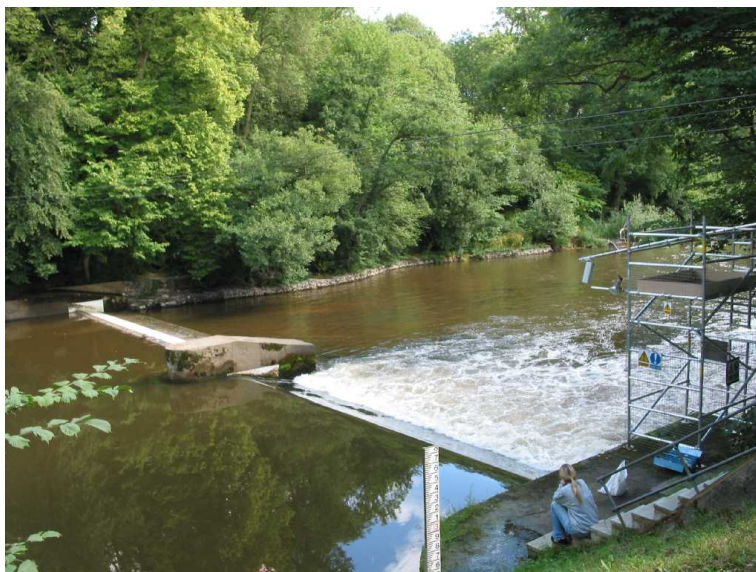
Figure 15: Manley Hall resistivity counter site showing the camera and lighting gantry
