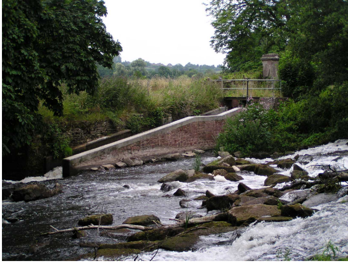
Figure 17: Larinier fish pass at Hampton Court on the River Lugg
