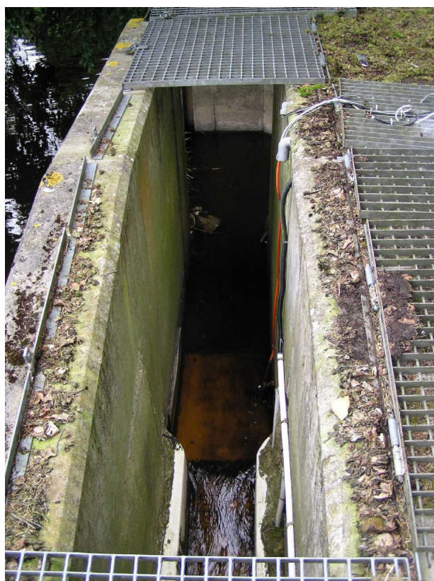
Figure 14: The North Warkworth pass. Cameras were deployed at the top of the pass
