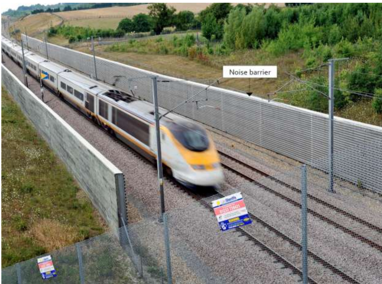
Figure 29: Photograph of an example of a noise fence barrier
