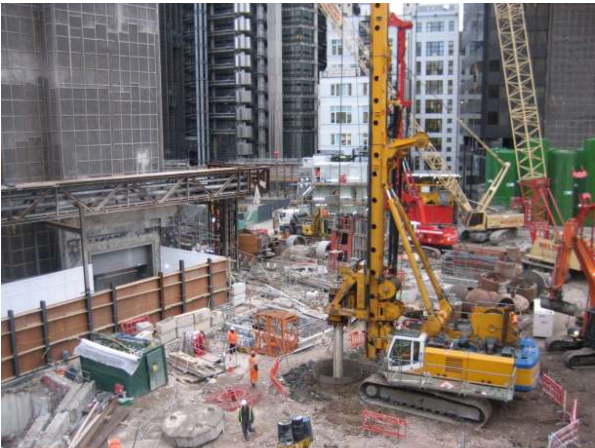
Figure 33: Photograph of an example of a piling rig
