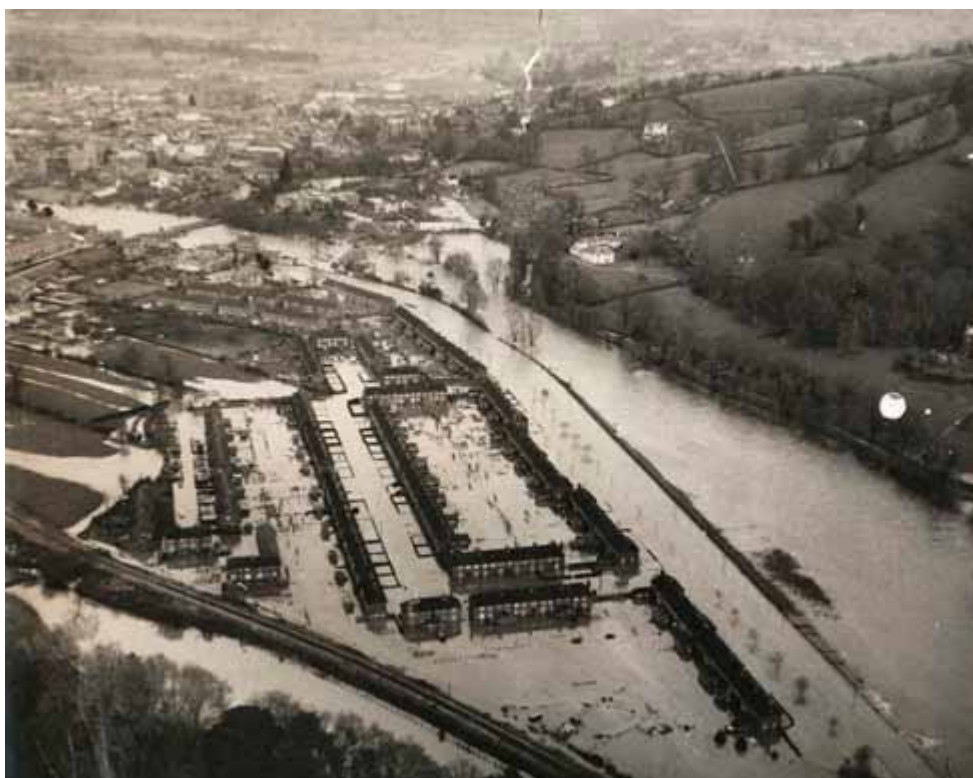
↑ Flooding on the south side of Tiverton
