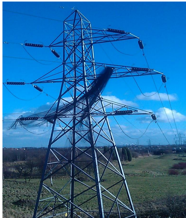
Netting caught on electricity pylon
