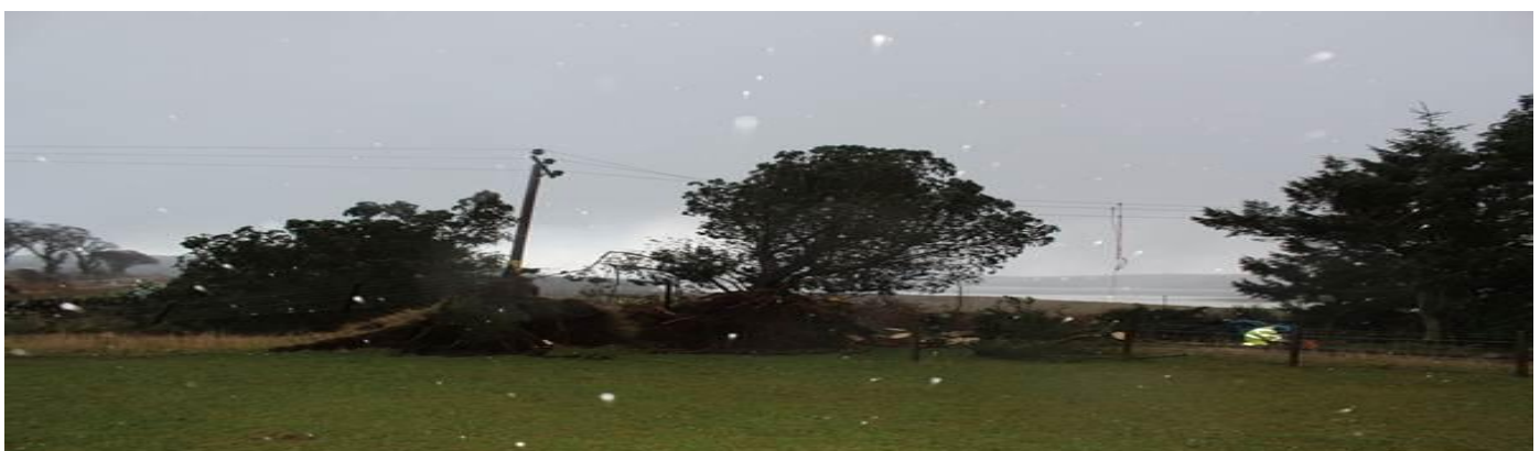
Trees uprooted on to power lines
