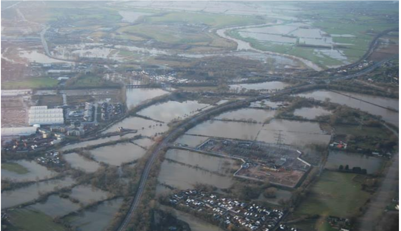
Electricity substation protected from surrounding flood waters
