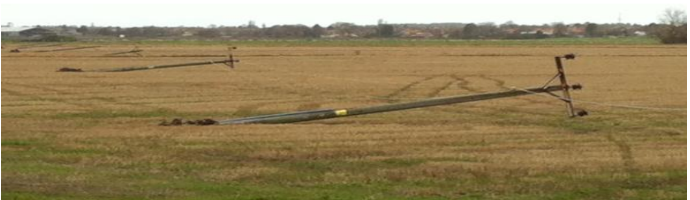
Power lines uprooted by extreme wind speeds
