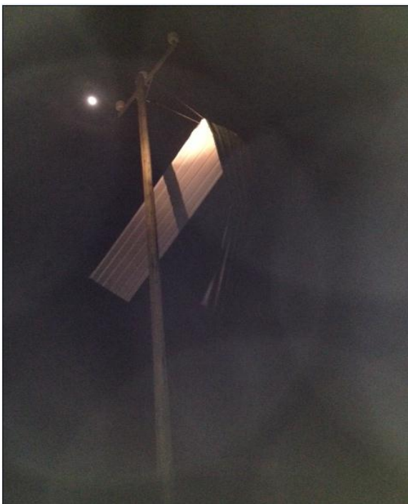
Metal sheeting blown on to power lines
