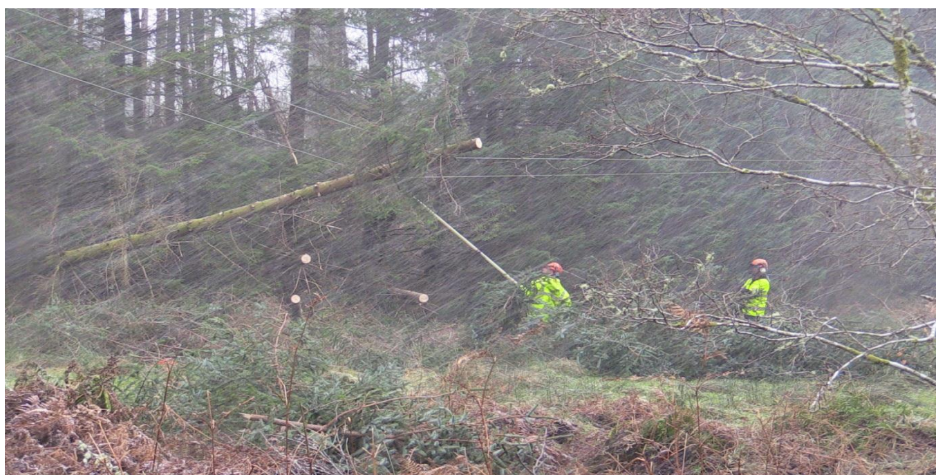
Engineers removing fallen trees from power lines in difficult conditions
