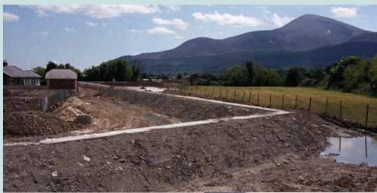
The scheme comprises 3,200 tonnes of steel sheet piles along with 3,000 cubic metres of reinforced concrete floodwall providing 3,300 metres of flood embankment along the riverbanks. In addition footbridges at 3 locations will be reconstructed and fisheries enhancement measures will be carried out.
