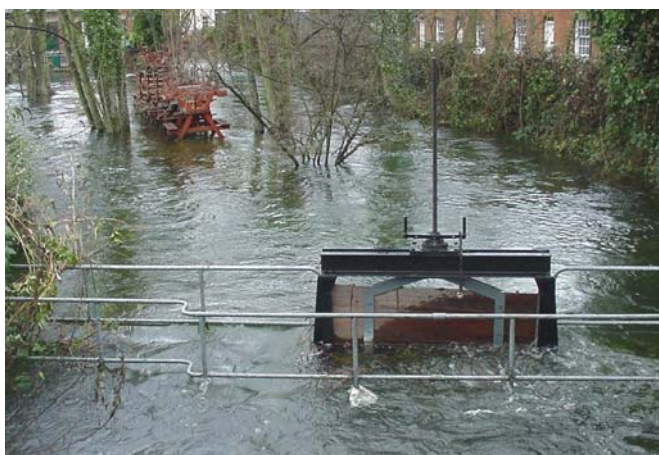
← Flood flows through Winchester.
