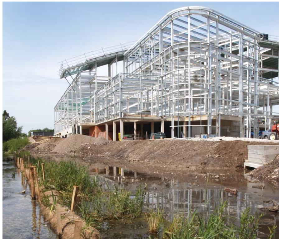
↑ River Anton river restoration.
