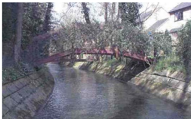
← Typical concrete trapezoidal channel in the Monks Brook.
