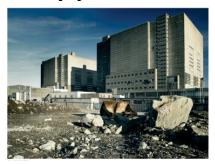
Trawsfynydd site is located in Gwynedd, North Wales. Electricity generation started in 1965 and ceased in 1991. Reactor defuelling was completed in 1995. The site continues to prepare for entry into Care and Maintenance planned for 2021, with the completion in 2009 of the recovery of bulk material from the Miscellaneous Activated Components (MAC) vaults and the relocation of the boiler sections.
