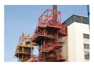
In March 2010, work to strip asbestos cladding from the heat exchangers, turbine halls and associated plant at Calder Hall was completed. The project, which has taken over five years, has seen the removal of 2,300 tonnes of asbestos cladding under extremely difficult working conditions and is considered to be the largest of its kind in Europe. Furthermore, this deteriorating asbestos insulation presented the highest conventional safety hazard across the NDA estate.
