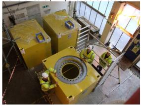
Also at Dungeness, we have seen encouraging results from a trial of new self-shielding 'ministores' (pictured above) suggesting that these could be used more widely to bring significant reductions to the cost of decommissioning.
