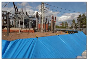
Temporary demountable flood barrier protecting the National Grid switching station in Walham, Gloucester, the day after the flood inundation in July 2007 (Courtesy of Geodesign Barriers Ltd).
