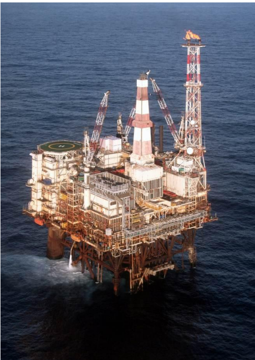
Figure 4: BP's Magnus Platform - a major gas injection EOR project in the North Sea.
