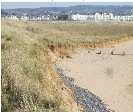
Plate 3.8: Eroded dune cliff and exposed gabions on Dawlish sand spit, view to north-east (FCRMU17)
