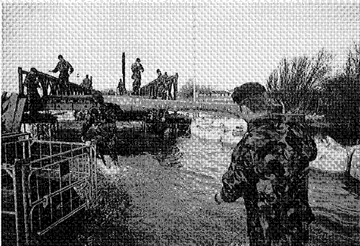
9(Para)Sqn Royal Engineers constructing a Bailey bridge at Chichester
