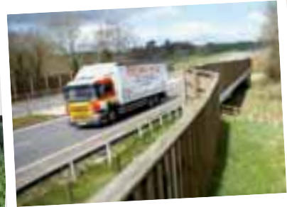
The villages of Wadesmill, High Cross and Colliers End now have a new bypass, reducing the volume of traffic traveling through the villages by more than 85%
