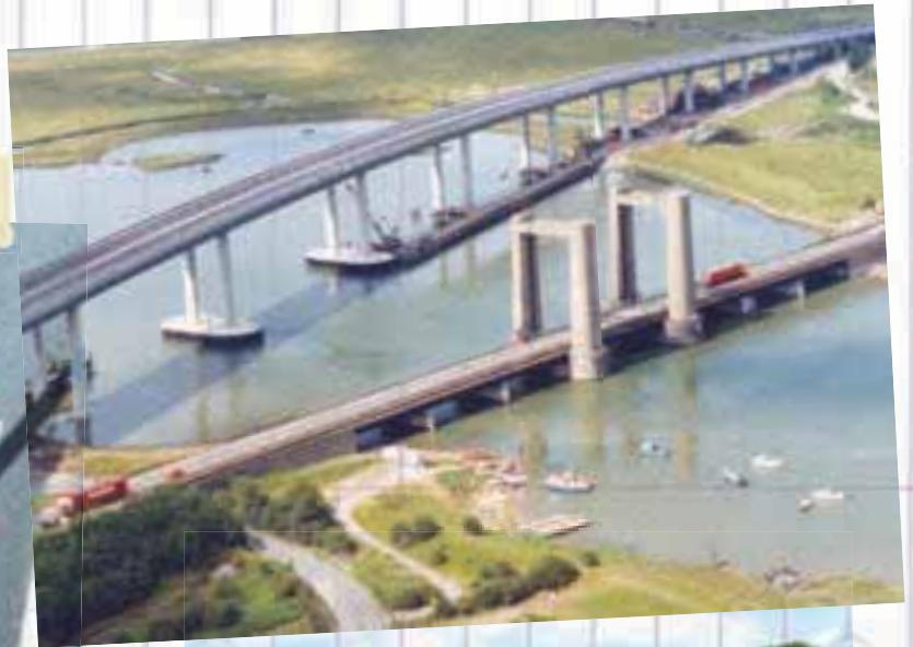
The A249 Sheppey Crossing. (Photo courtesy of Carillion)
