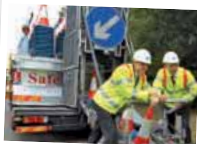
New cone laying machine
