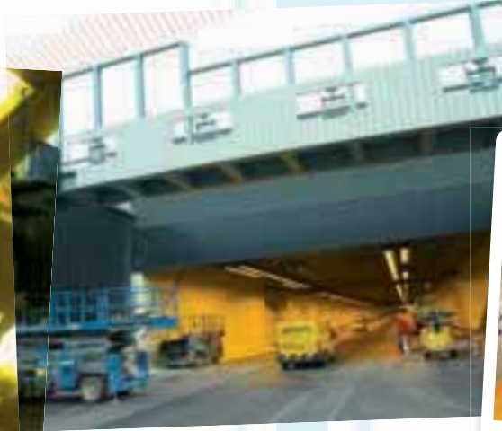
M25, Jct 25 Holmesdale Tunnel.
