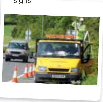
Highways Agency signs being positioned on M6 Junction 35 to 42
