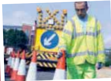
Road worker laying cones
