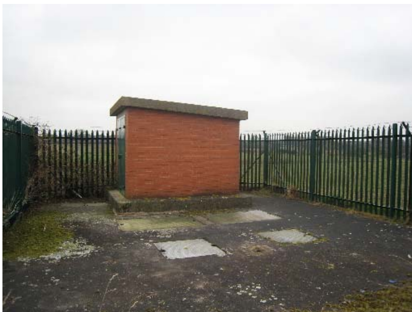
Figure A8.1 Highbridge pumping station
