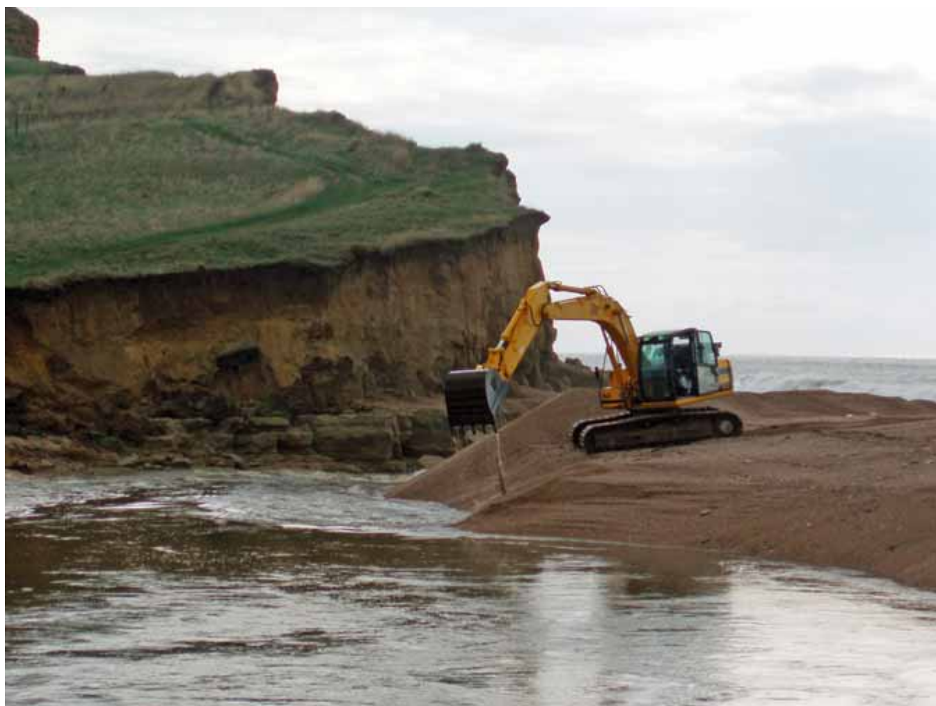
↑ Repairing erosion at Burton Bradstock, where the River Bride flows into the sea, in October 2006
