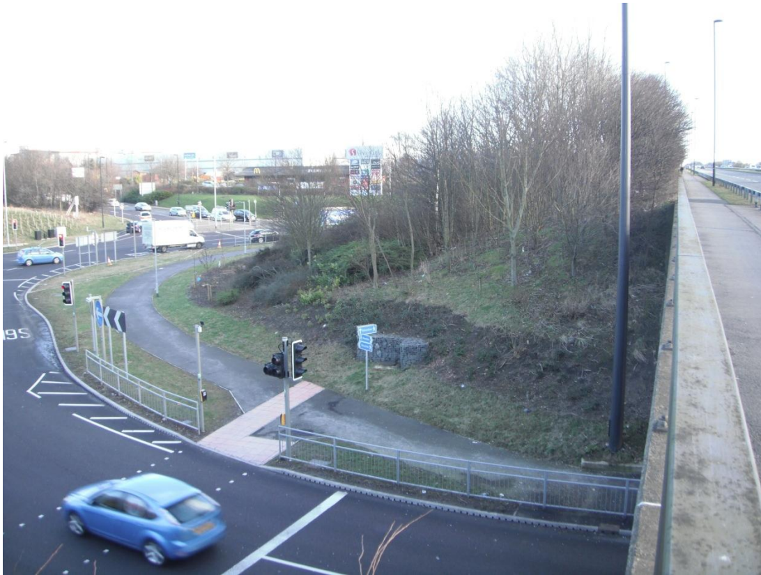
Silverlink Junction taken from the A1058 Coast Road
