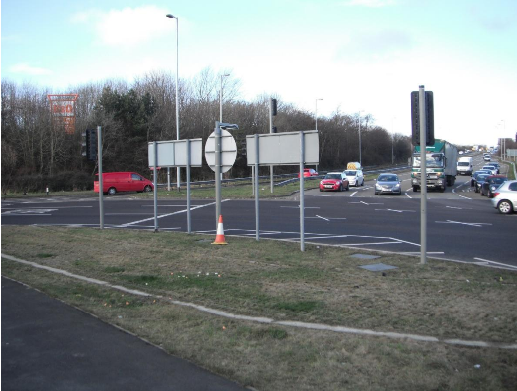
A19(T) North looking away from the Junction
