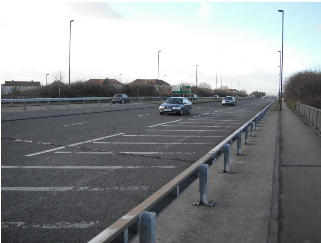
A1058 Coast Road Looking West
