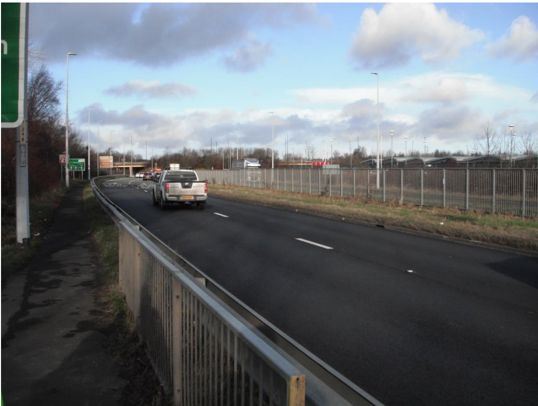
A19(T) South looking towards the Junction
