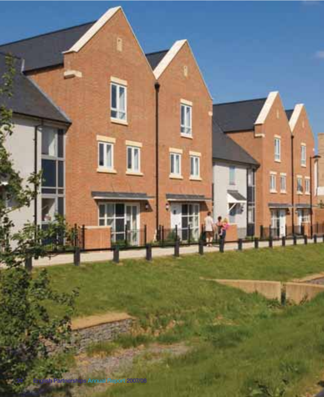
Sustainable urban drainage system (SUDS), Upton, Northampton.
