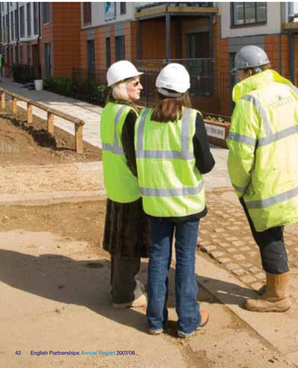
Construction at the Design for Manufacture site, Upton, Northampton.
