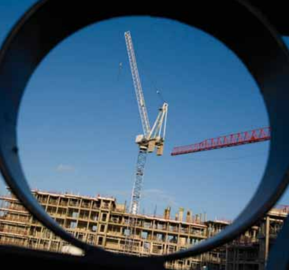
Left: Construction works at Wolverton, Milton Keynes.
