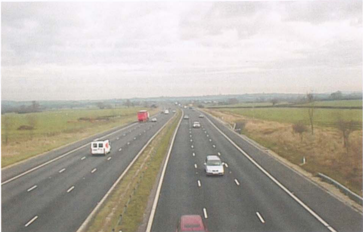
Photo 1 View of monitored carriageway - looking east
