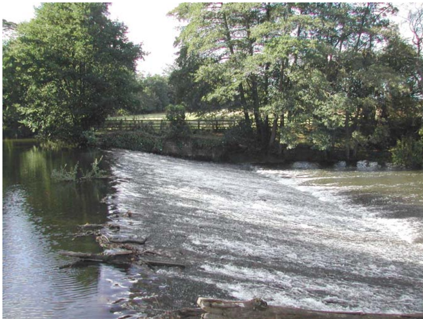
Figure 2.5 View of disused mill weir that marks the intersection between section B and section C. The photograph was taken during summer base flows and shows the shallow depth over the crest and downstream face across the full width (about 34 m) of the weir.
