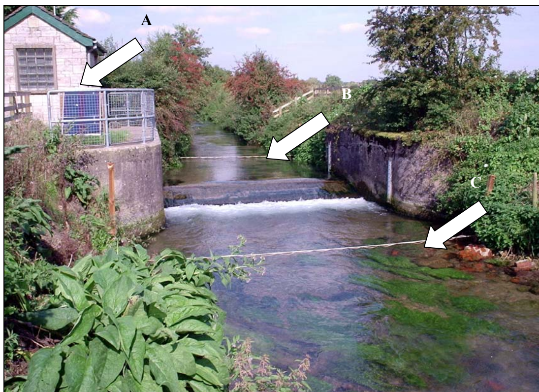
Figure 3.3 Costa Beck Crump gauging weir with PIT detection equipment. Arrows show: A, solar panel power supply; B, upstream antenna; C, downstream antenna.
