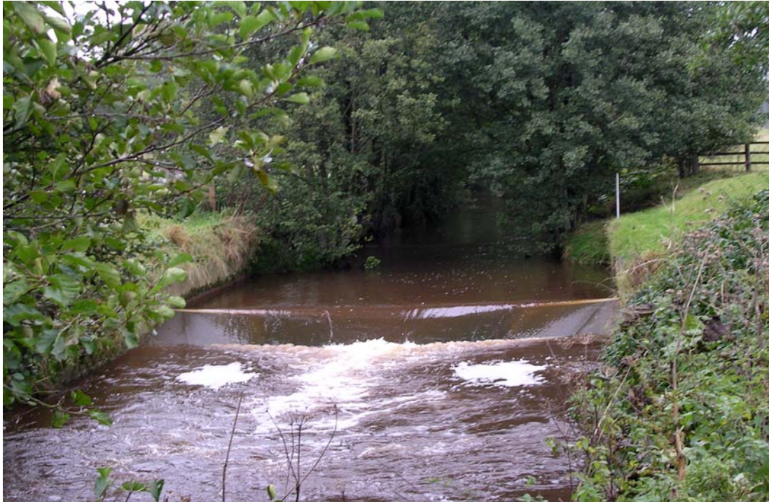
Figure 3.4 Kirkby Mills Flat-V gauging weir on the River Dove during elevated flow conditions. Upstream antenna is about 20 m upstream of weir beneath trees (not visible), and downstream antenna is 5 m downstream from where photograph was taken.
