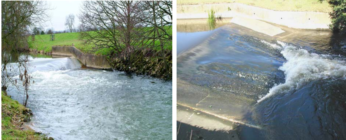
Figure 2.4 Ness Flat-V flow-gauging weir showing an oblique view from downstream at moderate winter flows (left panel) and a close-up view of the downstream weir face at low summer flows, which highlights the shallow water on the weir face, hydraulic jump at the base and the flow eddies on each side (right panel). The weir is approximately 12 m wide.
