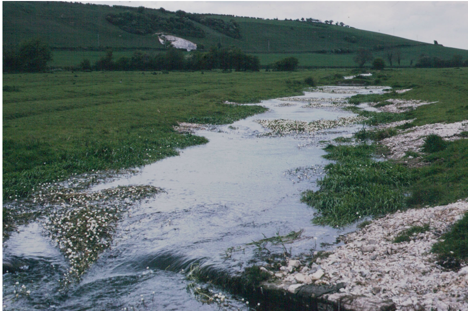
Figure 40 Series of low profile, upstream 'V' current-deflectors, scouring pools and stimulating Ranunculus growth on faster-flowing intervening riffles, Devil's Brook, Dorset
