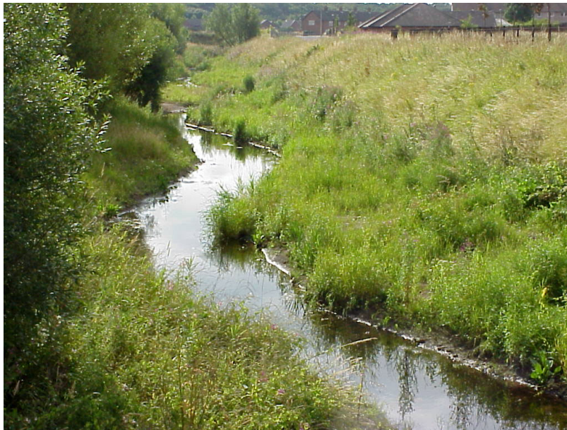
Figure 50 Channel narrowing creating a two-stage channel
