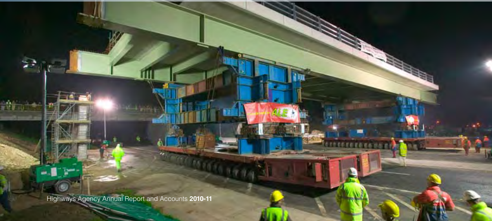
Installation of a pre-fabricated steel composite bridge deck
