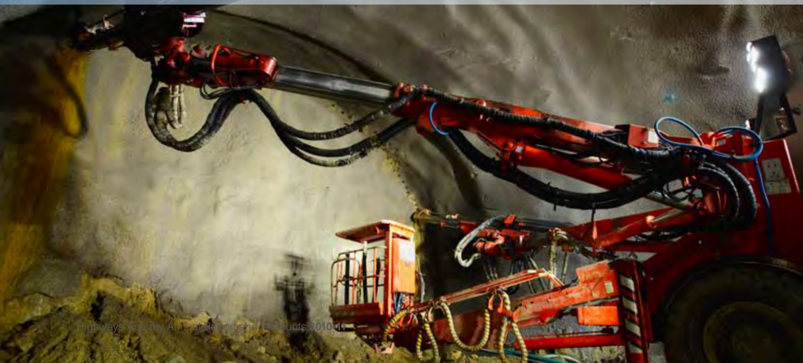
Excavation of the tunnels at Hindhead
