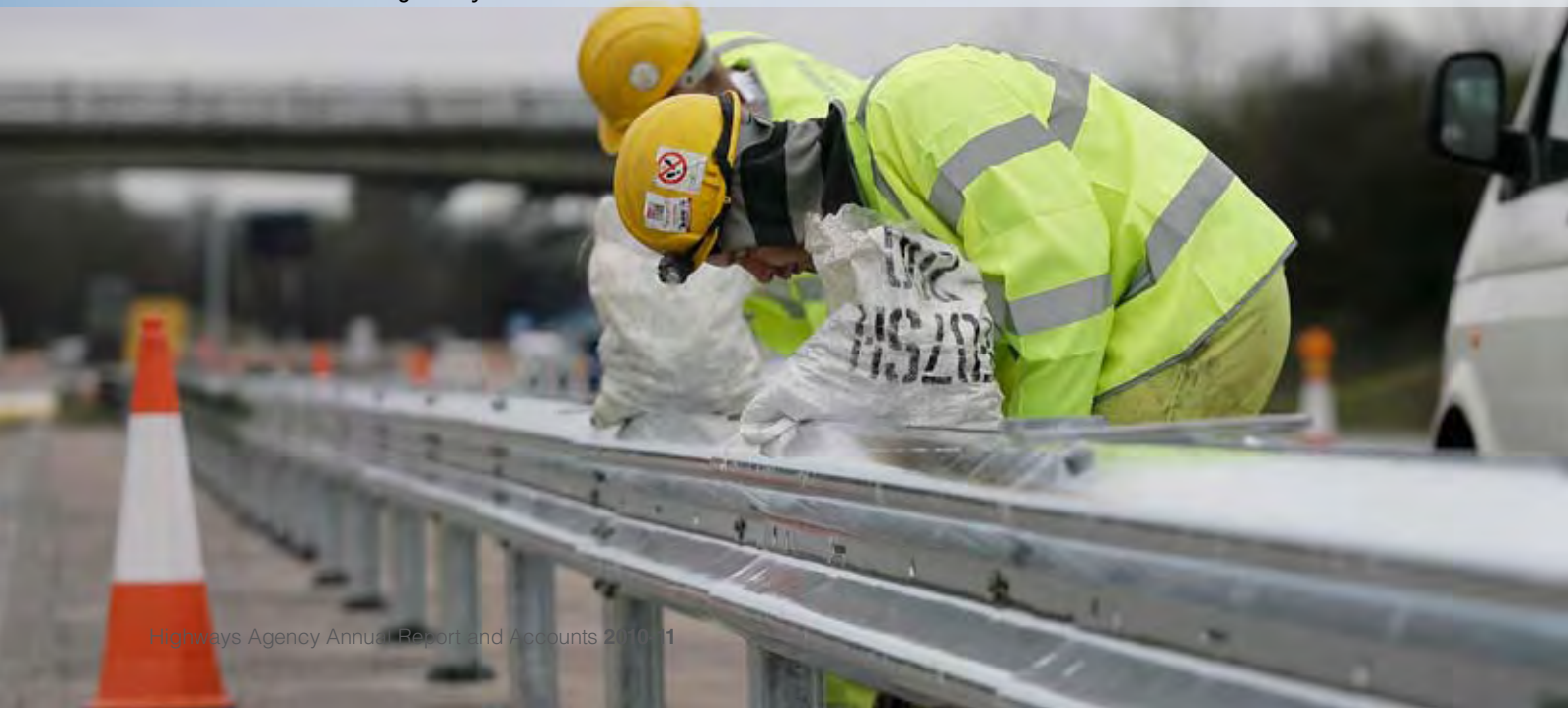
Road workers installing safety barriers
