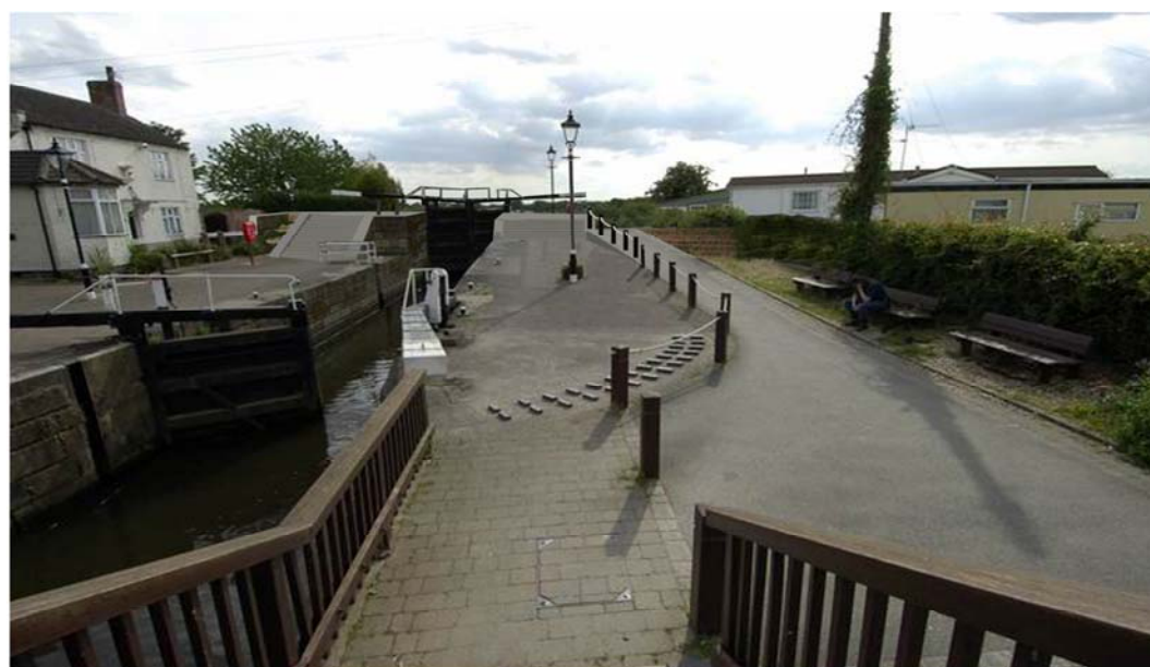
Plate B7.13 'Photosketch' Visualisation showing Beeston Locks Re-Grading (refer to Plate B7.12)
