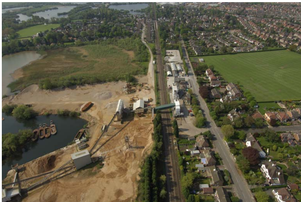
Plate B7.5 Aerial View of the Cemex Works site (Reach 10)
