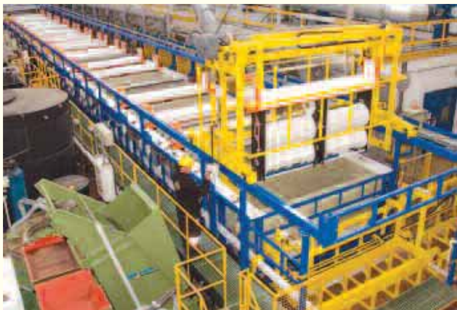
The new nickel-plating plant, rebuilt after a damaging fire, is a world-class facility of which we are justifiably proud.
