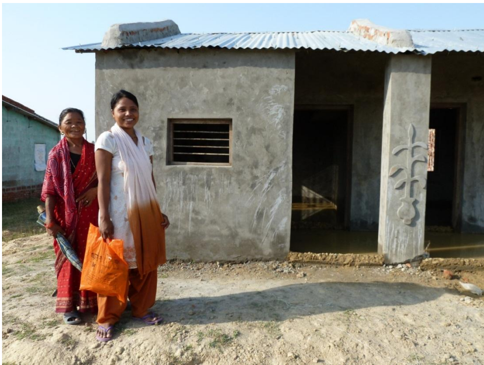
New owners next to their near-completed house in Kohalpur, Nepal. Photo credit: CLIFF
