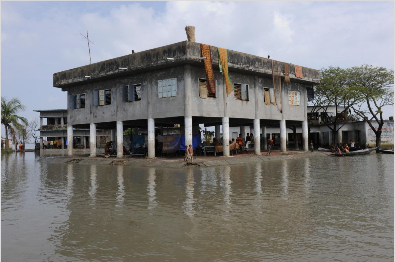
Cyclone shelter built under the DFID supported Bangladesh Climate Change Resilience Fund. Photo credit: DFID-Bangladesh
